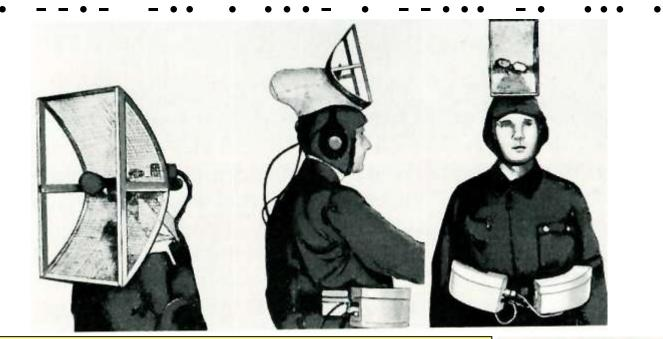
Telefunken FuMB 33 *Liliput 1* body-worn detector (2.5-3.75 GHz) for use in small craft without on-board power. The belt-worn amplifier was fragile and had poor sensitivity. Due to the 50° beamwidth, the operator "scanned" by constantly turning his head back and forth. Deployed in September 1944; 300 units built. Also issued to U-boats.
