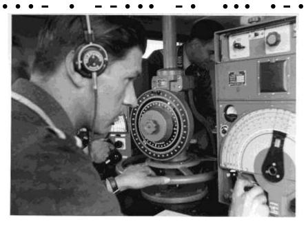
Interior: Operator at EP2a RX (75 kHz - 3.3 MHz).
