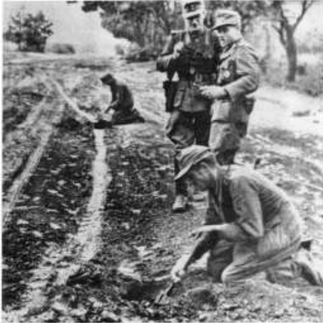
Not only were enemy mines removed, but their own were laid. Engineers prepare a quick barrier, Italian front, 1944.
