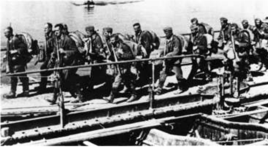
A company with packs, rifles carried as in World War I (rarely done in World War II), crosses a finished military bridge shortly before the ramp section.
