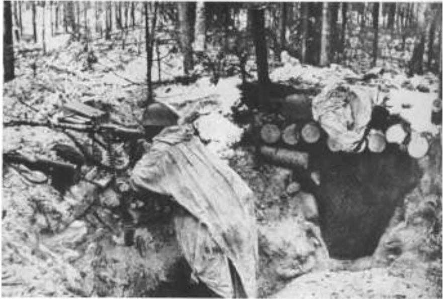
The front line — a trench with a dugout.
