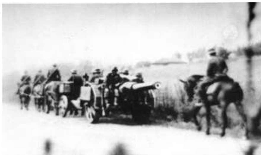
The 150mm heavy field howitzer, carried dismantled in two horse-drawn wagons, the barrel wagon shown here (western campaign, 1940).
