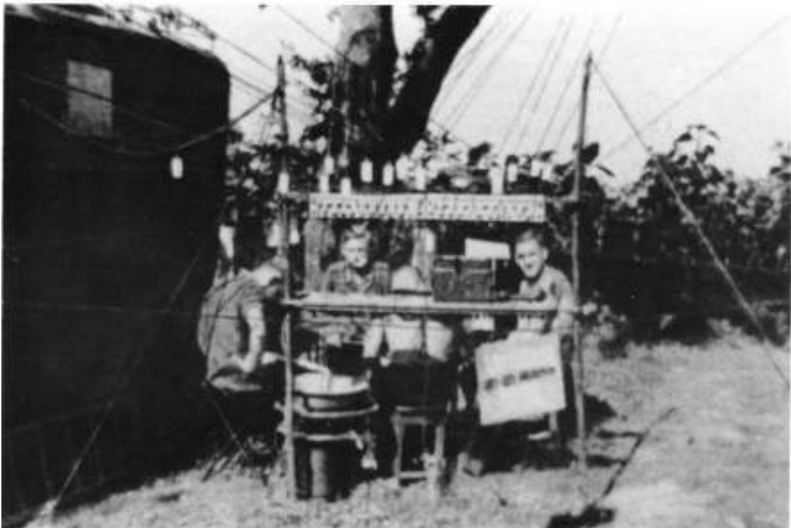
The division switchboard with lines coming in; at left a big telephone truck.
