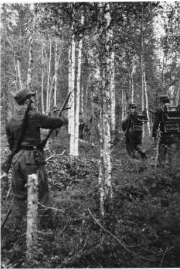
Putting up telephone lines in the forests of Karelia, at right the men with the cable drums on their backs, at left the soldier with the pole for high work, eastern front, 1942.
