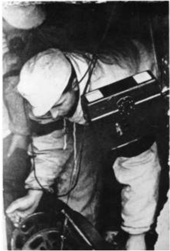
A field telephone is hooked to the wires in a bunker.
