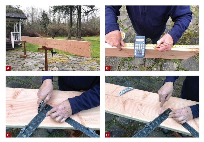
Figure 3. The author places his stringer stock on edge with the crown up (A) to mark the diagonal increments, using the plus/equals function on his calculator to determine the exact distance of each increment from his starting point (B). The increments guide the placement of the framing square as he marks the notches with a utility knife (C). Highlighting the layout lines with a pencil makes them easier to see when cutting the notches (D).
