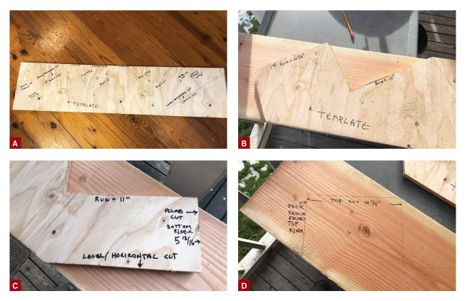
Figure 2. After calculating the unit rise and run following the steps shown in the drawing on the facing page, the author lays out a few treads and risers on scrap plywood ripped to the width of the stringer stock (A). He uses this template to check the fit at the top (B) and bottom (C) of the stairs prior to laying out and cutting expensive stringer stock (D).
