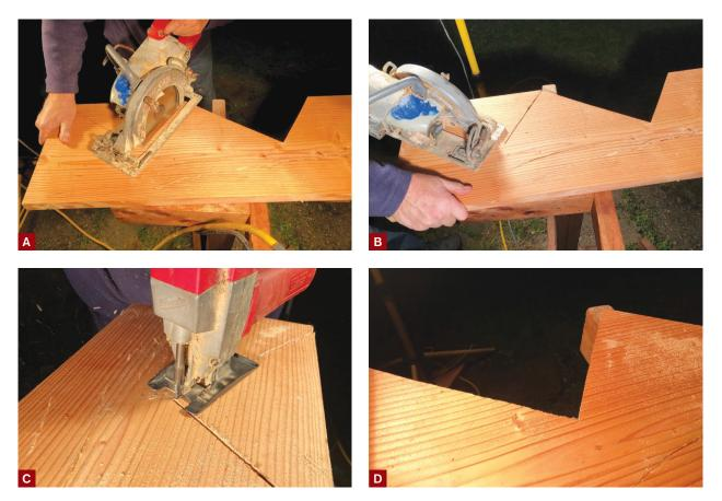
Figure 4. To avoid overcutting the notches, which would weaken the stringer, the author starts the cuts with a circular saw (A, B), and finishes the cuts with either a handsaw or a jigsaw (C). Marking the diagonal increments on the stringer before laying out and cutting the notches ensures that tread and riser dimensions vary by no more than  $1/_8$  inch (D).
