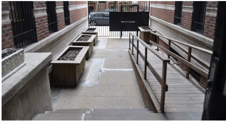
An accessory ramp installed at the enclosed areaway of a large apartment building.
