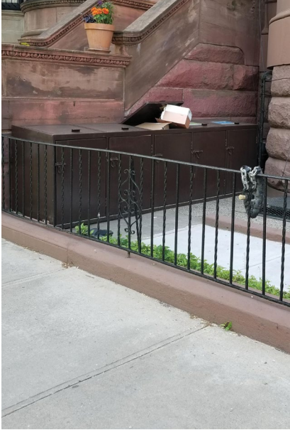
A garbage enclosure with a compatible finish and color attached to non-historic areaway paving.
