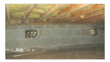
Insulation must maintain permanent contact with underside of subfloor
