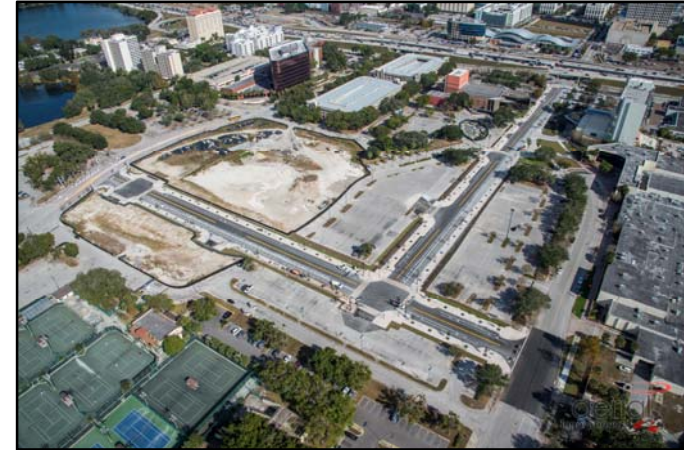
Aerial of LYMMO Lime Line in Creative Village
