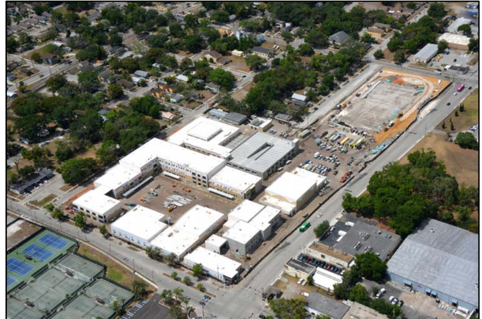
OCPS Academic Center for Excellence – (Aerial April 10, 2017)
