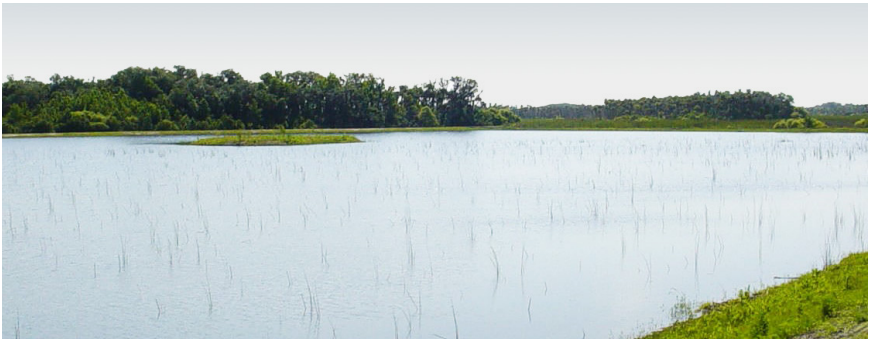
The renovated wetland cell is re-flooded.
