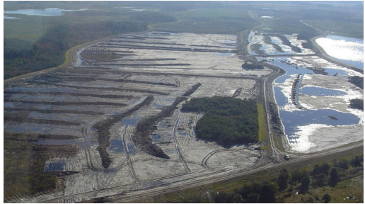
Muck is piled into rows and allowed to dry out
