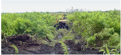
Bulldozers begin to pile up the vegetation and accumulated muck
