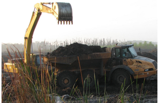
The muck is loaded into trucks and removed from the cell.
