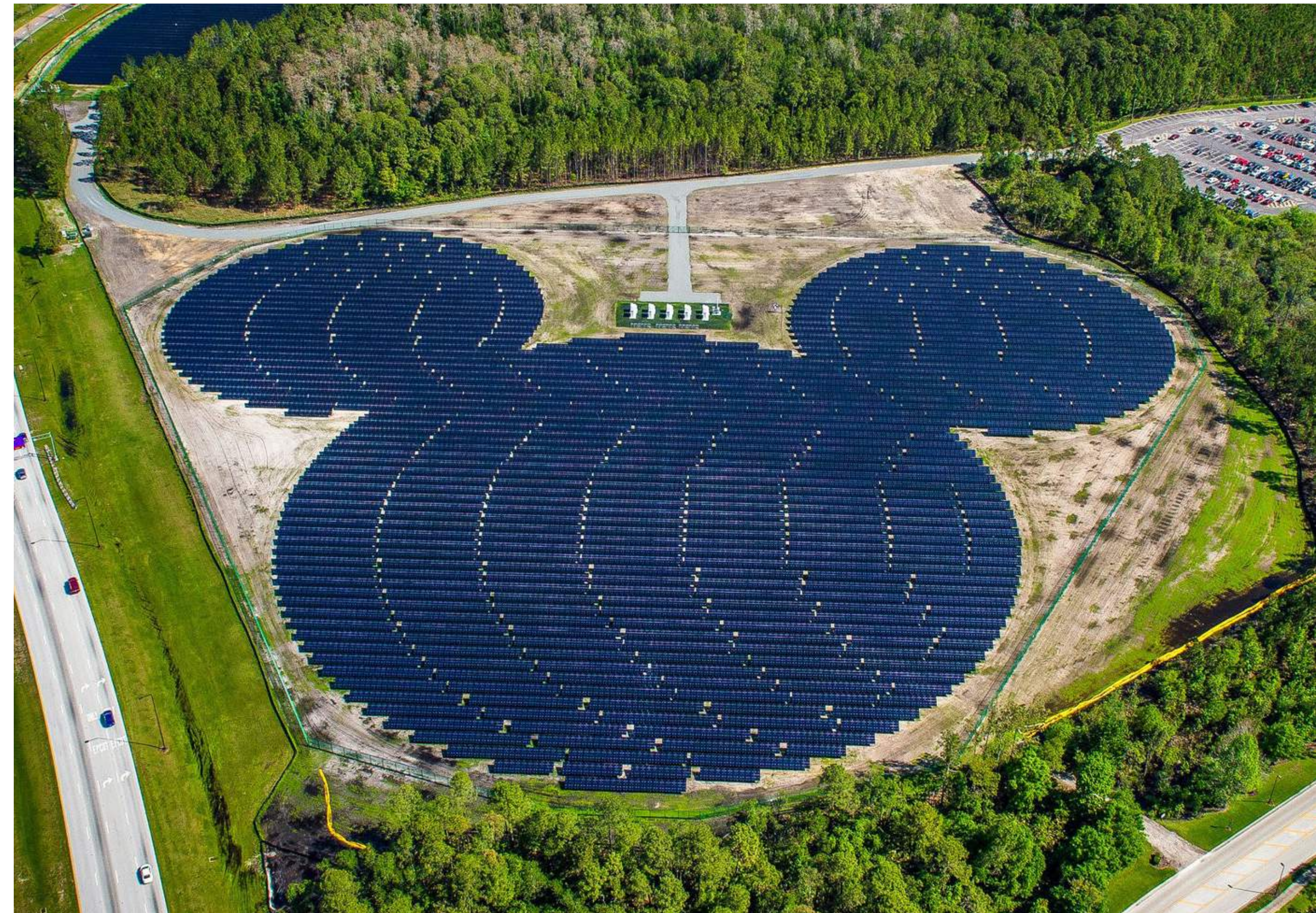
Solar array at Walt Disney World
