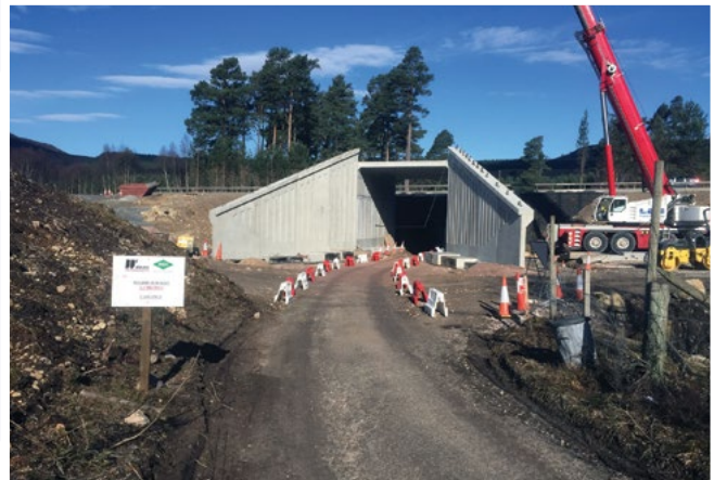
New underpass at Lower Milehead
