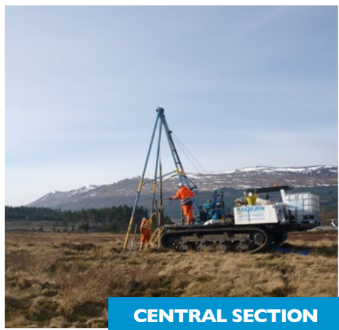
Preliminary ground investigation works underway
