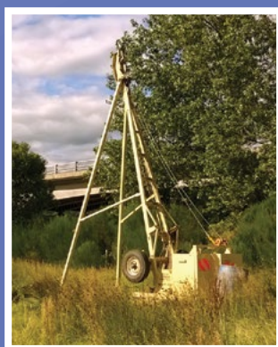
Cable percussion borehole at River Tummel Crossing, Pitlochry – advanced ground investigations, 2015
