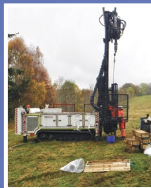
Sonic borehole, Pitlochry – advanced ground investigations, 2015
