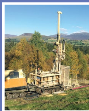
Rotary borehole north of Shierglas Quarry – advanced ground investigations, 2015
