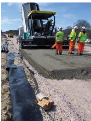
Laying the new road surface
