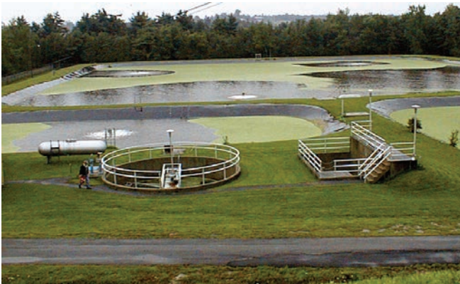
Aerated lagoons are secondary treatment processes.
