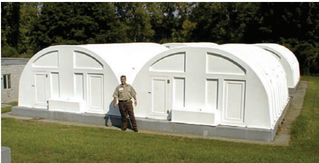
Rotating biological contactors (Secondary Treatment).
