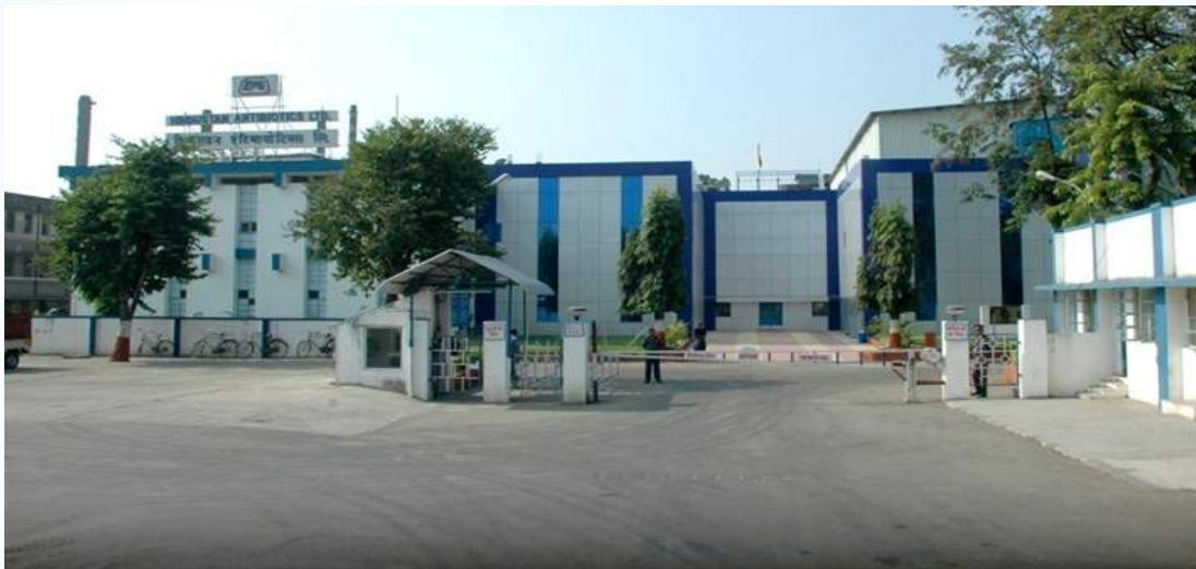
HAL- Building front view of Cephalosporin Plant
