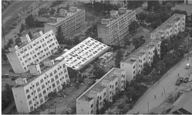
Liquefaction (Niigata, Japan 1964)
