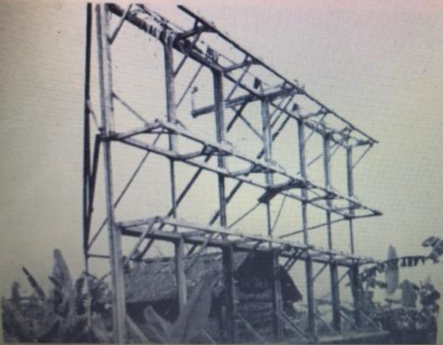
The Imperial Japanese Navy sent nearly one-third of its long-range land-based early warning radar units to defend Rabaul. This unit was one of two installed at Tomavatur Mission, 2 miles southeast of Vunakanou. (AC)
