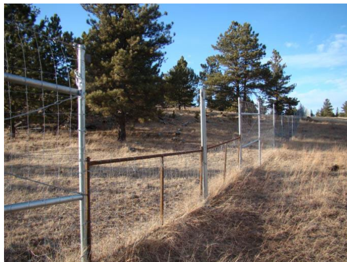
Figure 14. Photo of double wide elk jump gate in lowered position (Photo Credit: Wind Cave National Park).
