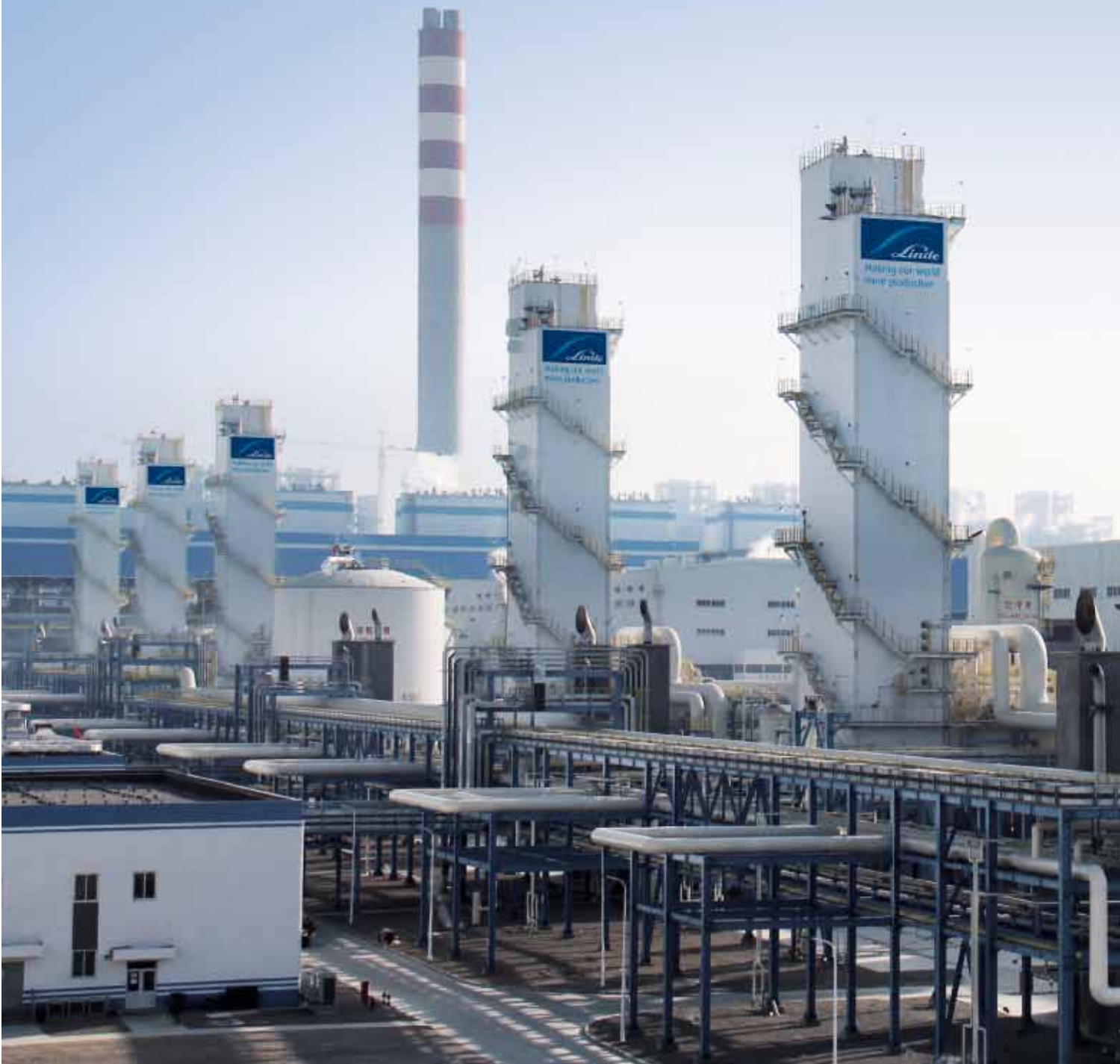
Air separation units near Yinchuan, China.
