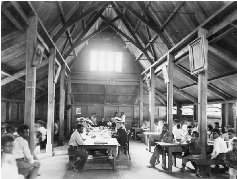
Figure 4.10: Interior of the St Barnabas College dining room, Norfolk Island.
