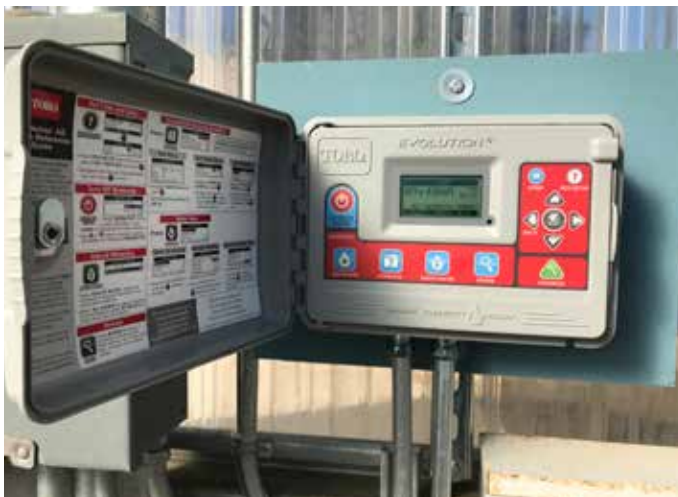
FIGURE 22. Typical low-cost irrigation controller capable of running multiple schedules programmed to meet different crop needs.
