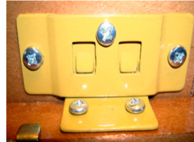
Slide Locking Plate Over "L" Bracket
