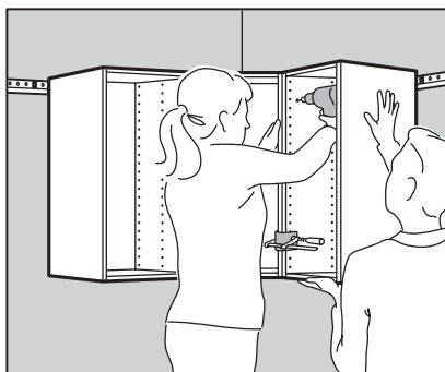
Hang the corner cabinet first and secure by tightening the screws. Hang the remaining cabinets and connect them with the included screws. Wait to tighten the screws until the base cabinets are in place and you can ensure alignment.
