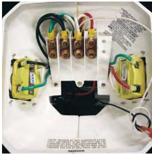
Copper Busbar with Ratings up to 140 A
