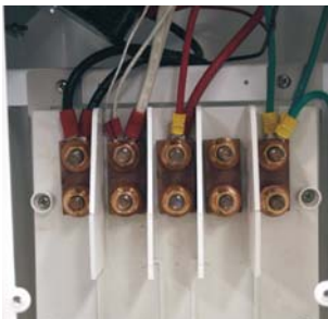
Copper Busbar with Ratings from 250 to 500 A
