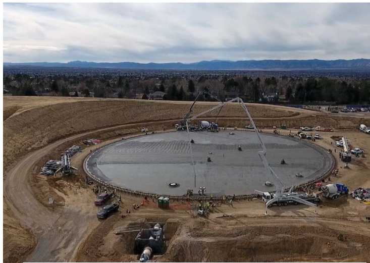
Hillcrest Storage Tank Replacement
