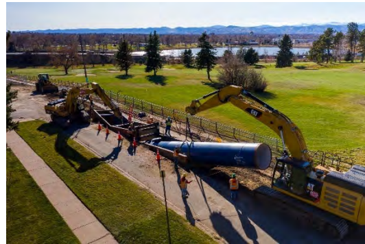
Construction crews install a 50-foot section of steel pipe next to Willis Case Golf Course in northwest Denver. Large pipes are 66 inches in diameter and weigh 11,500 pounds.
