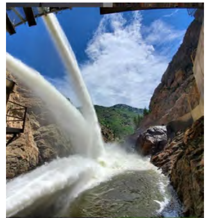
Strontia Spring's semi-annual ERDS flush, a 50-foot-long tunnel that is critical to dam safety.
