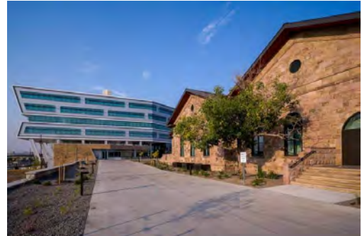
Operations Complex and Three Stones Building – October 2020
