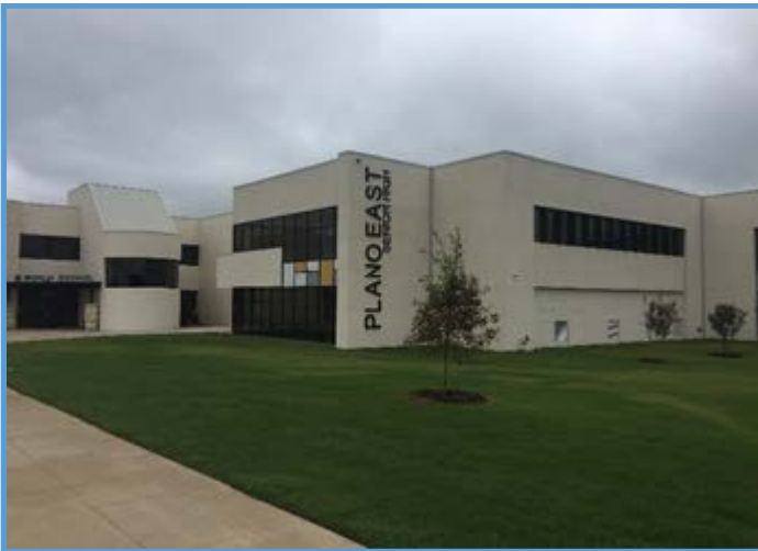
Plano East Senior High School, New Addition Exterior, September 2018
