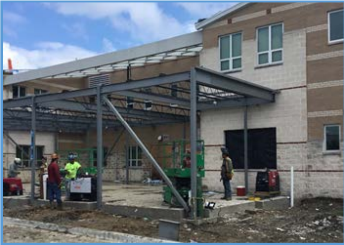
Jasper High School, Art Room Addition, September 2018
