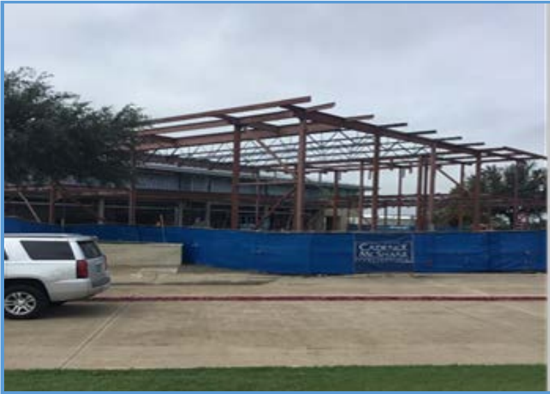
Robinson Middle School, Main Entry Steel, September 2018
