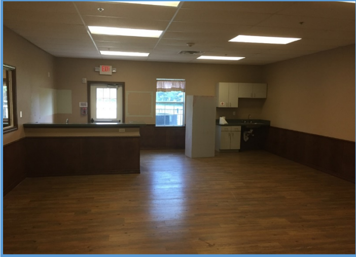
Employee Child Care 3, Interior Rooms under Construction, June 2018
