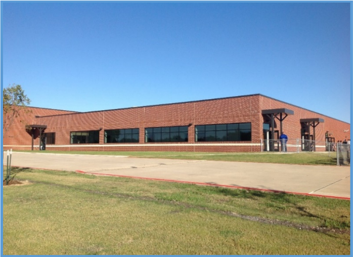
Guinn Special Programs Center, Classroom Addition, August 2017
