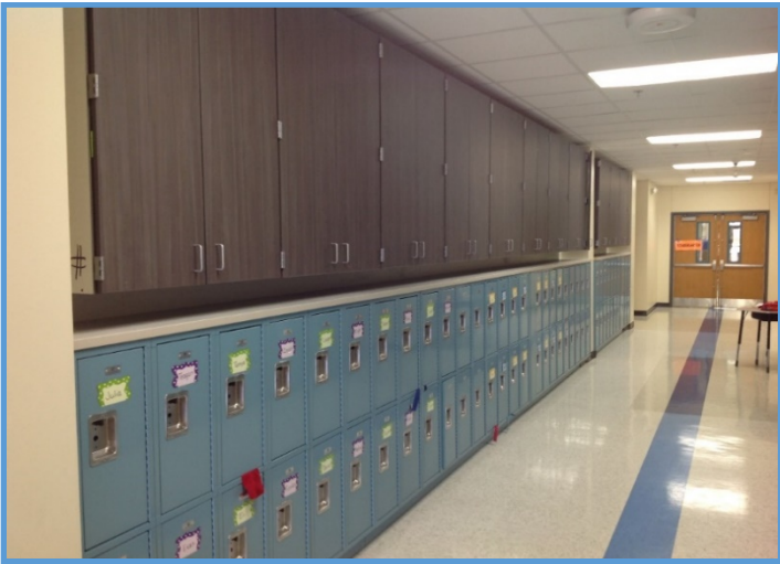
Rose Haggar Elementary School, Refurbished Classroom Pod, October 2017
