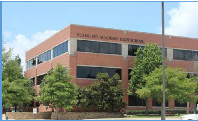
Academy High School Re-Brick, New Brick Veneer, October 2017
