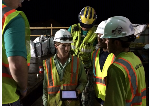
Interns participating in an early-morning concrete pour.
