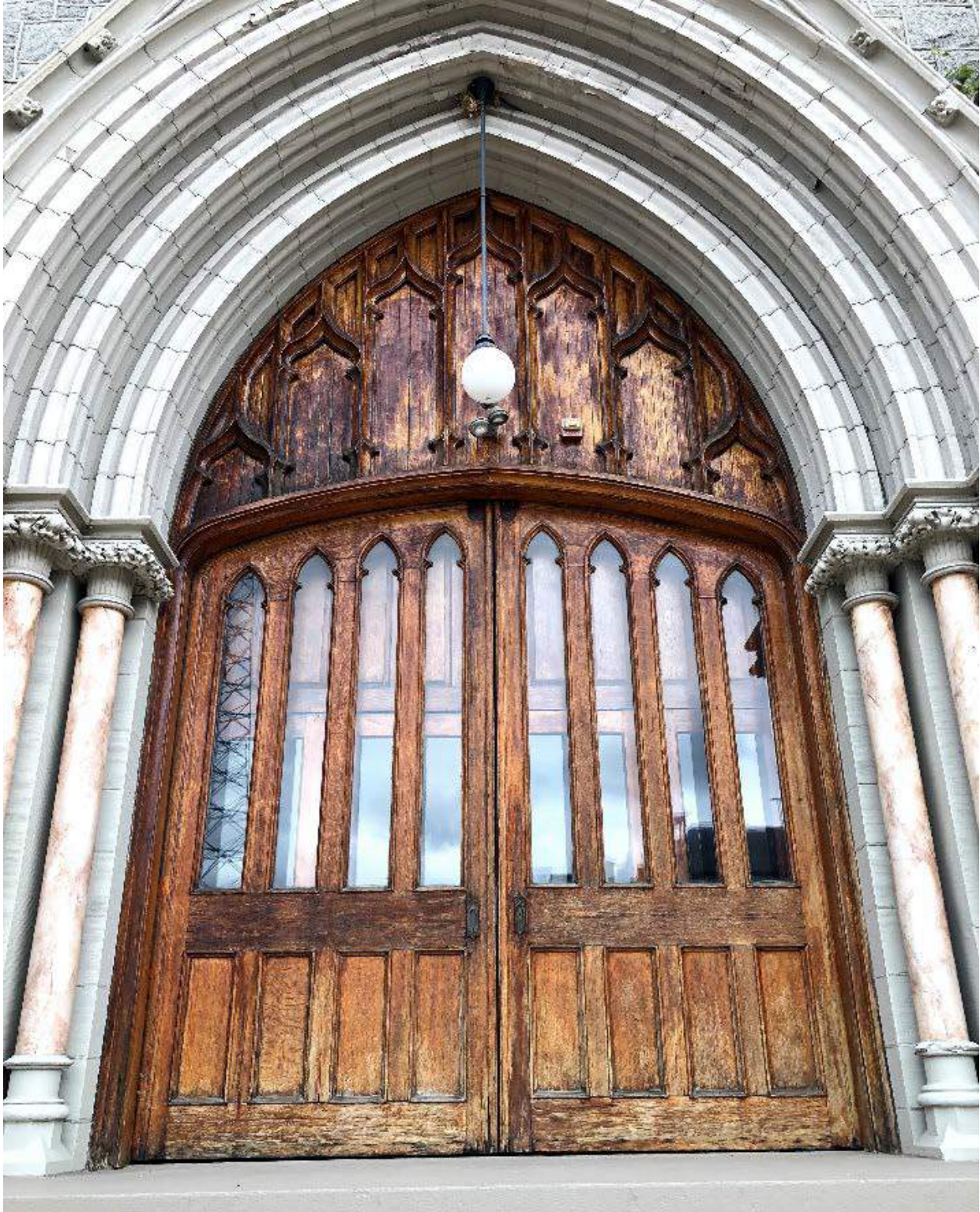
Figure 7. Detail of central door at south elevation. [Arielle Harris, September 2019]
