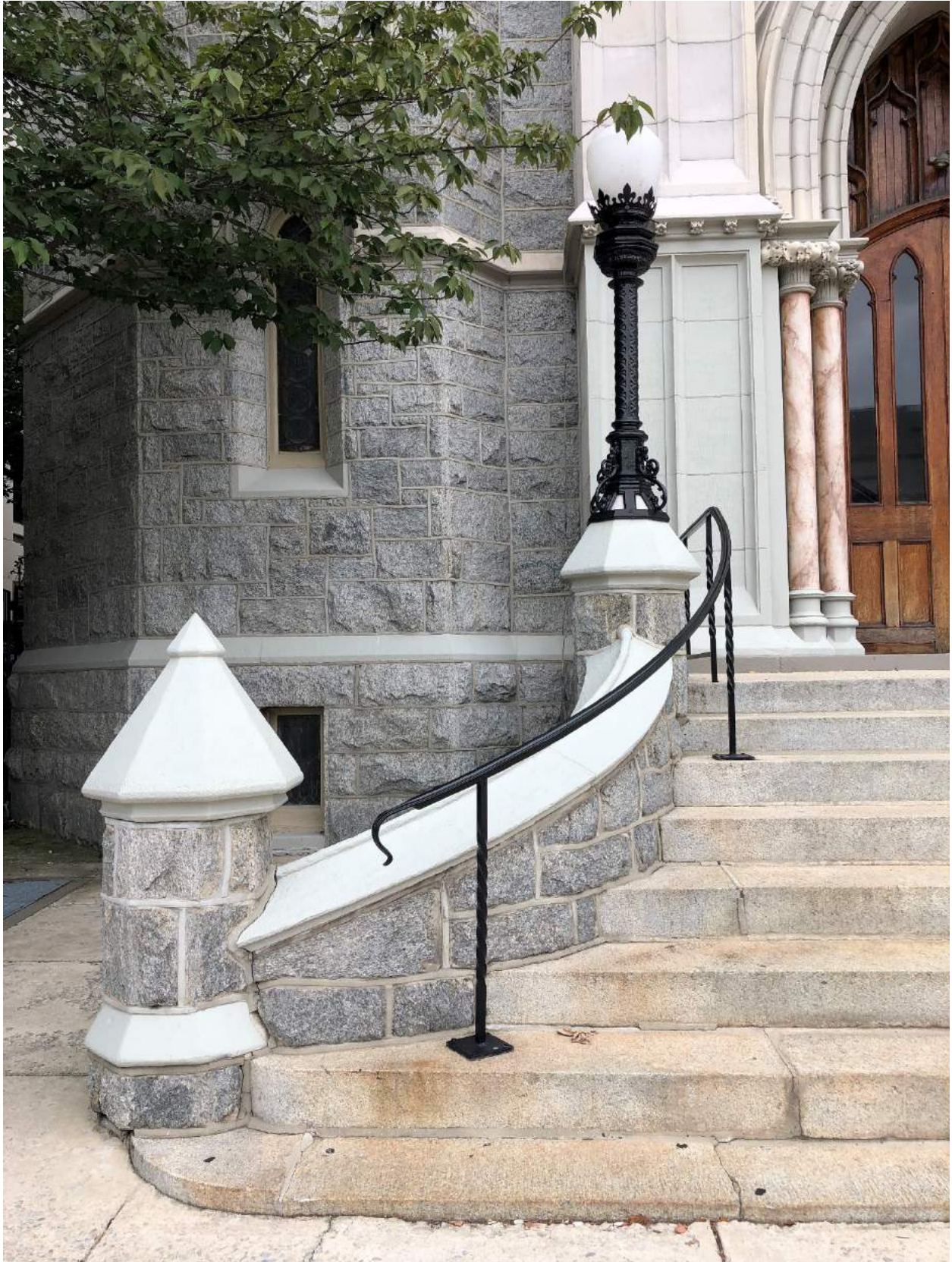
Figure 6 Detail of west stair rail and ornamental lightpost [Arielle Harris, September 2019]
