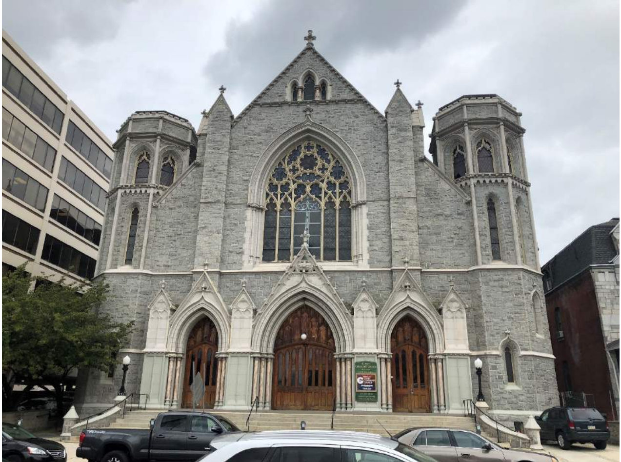
Figure 4. South (principal) elevation of New Tabernacle Baptist Church, now in use as Christ Community Church [Arielle Harris, September 2019]
