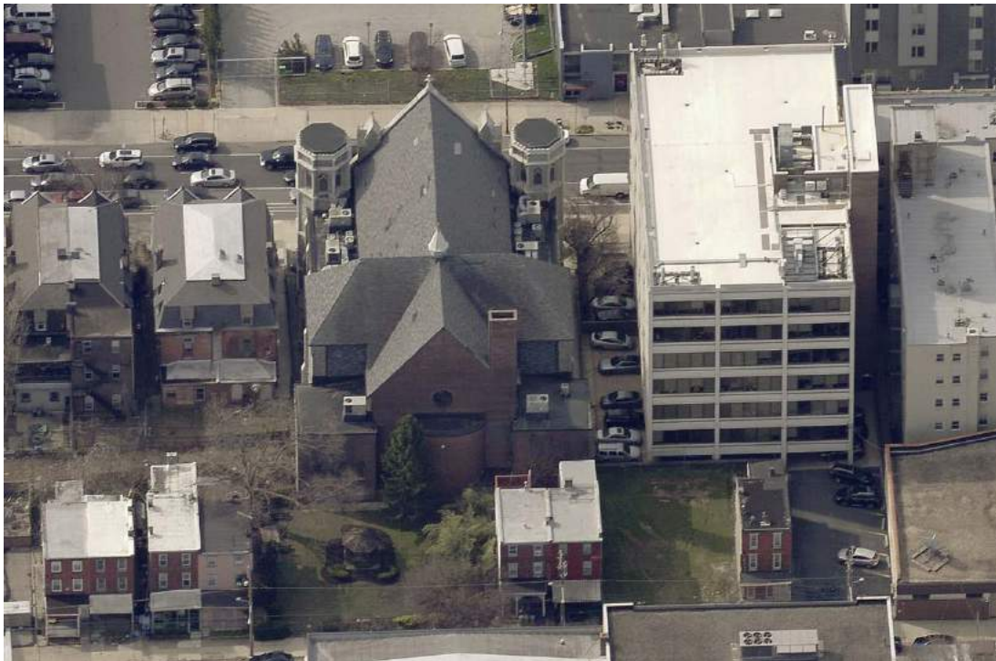
Figure 12. Oblique view looking south at New Tabernacle Baptist Church, providing a clearer view of the north elevation. [Pictometry]
