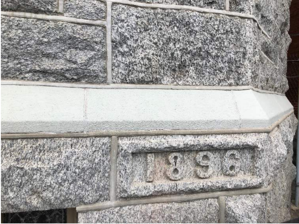
Figure 5. Detail of cornerstone at eastern tower. [Arielle Harris, September 2019]
