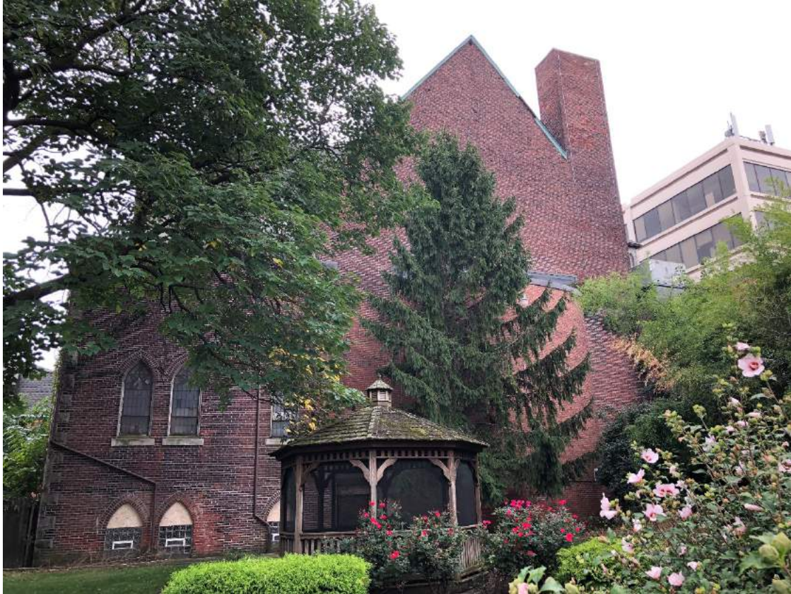
Figure 11. North elevation. [Arielle Harris, September 2019]
