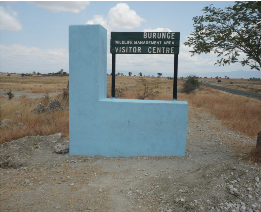
Fig. 1. Burunge Tourist Centre under construction. Photo by Gerson Mollle, 2011
