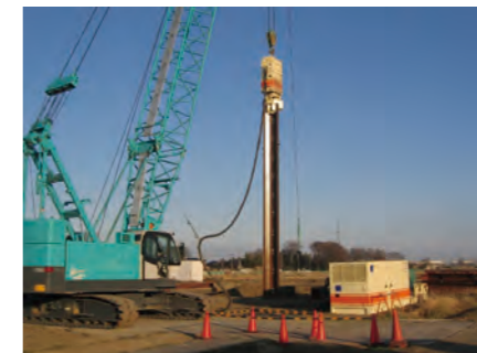
Case example of a repeated use test using a vibratory hammer
