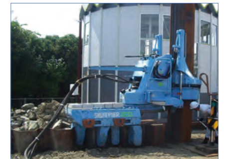
Case example of a repeated use test using a press-in machine
