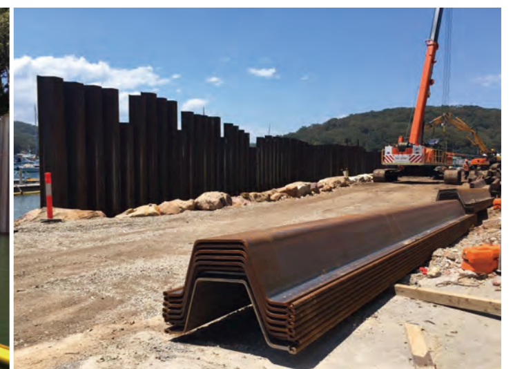
Hat-type Sheet Pile Church point seawall / Australia
