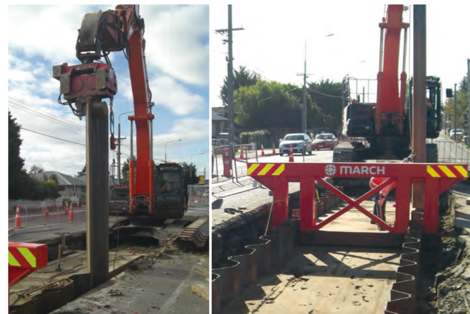
Hat-type Sheet Pile / New Zealand
