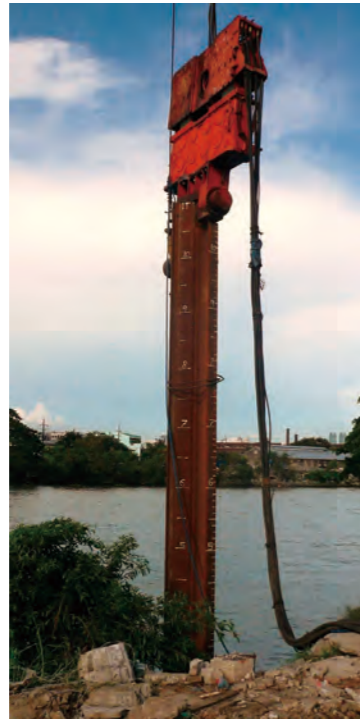
Driving of a Hat+H sheet pile
