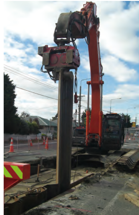
Driving of a Hat-type sheet pile
