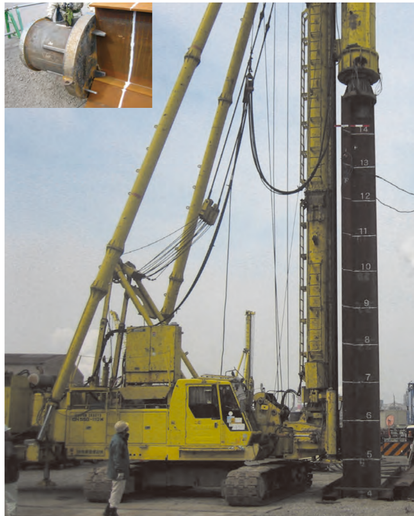
Driving of a Hat+H sheet pile
