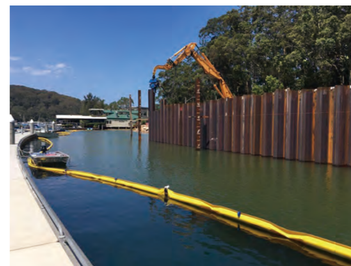
Hat-type Sheet Pile Church point seawall / Australia
