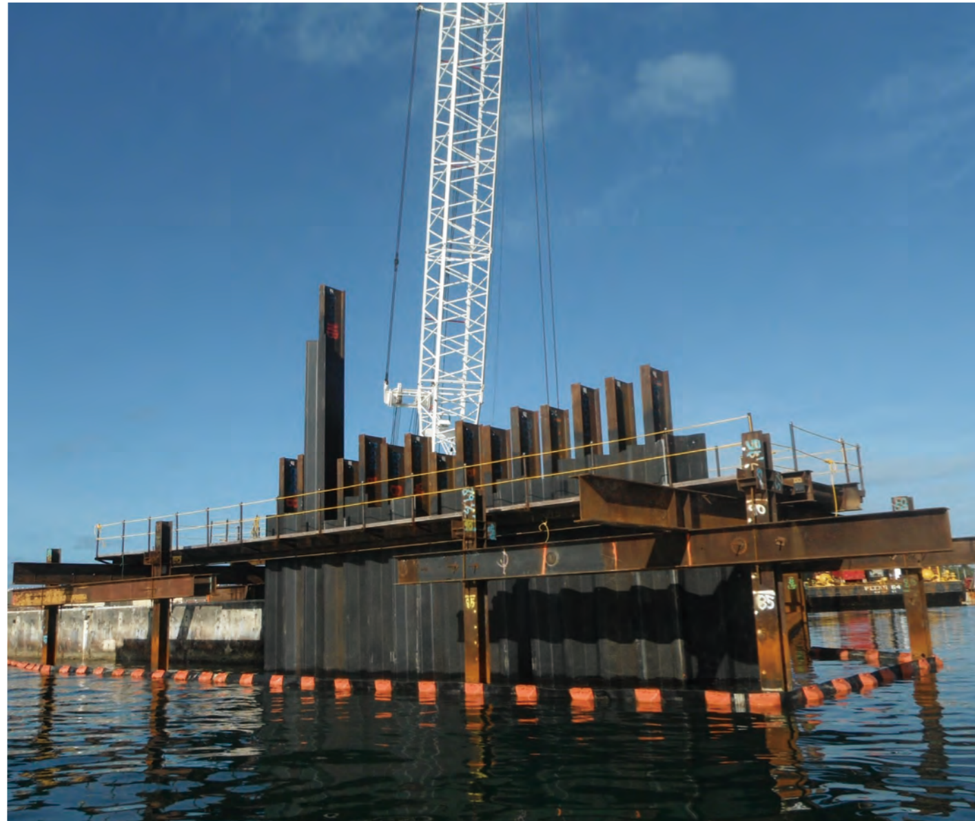
Hat+H Guam Apra Port refurbishment / USA
