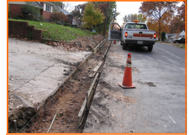
Curb forms being made ready for concrete
