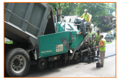
Typical asphalt paving operation
