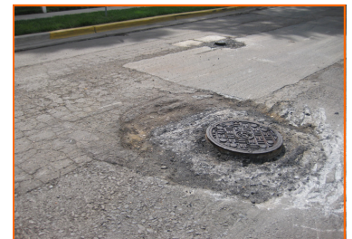
Utilities will be raised to meet new HMA
