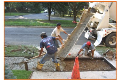
Pouring new concrete into forms
