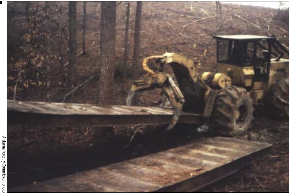
Installation of one of the types of temporary bridges that can be used.
