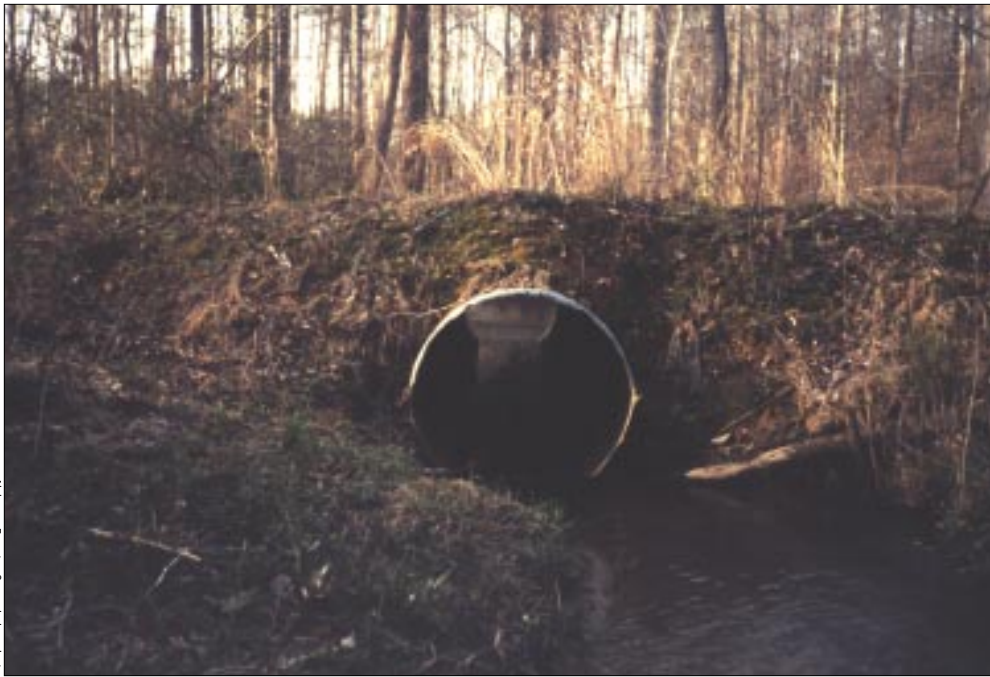
A permanent culvert of adequate size has been installed on this forest access road.
