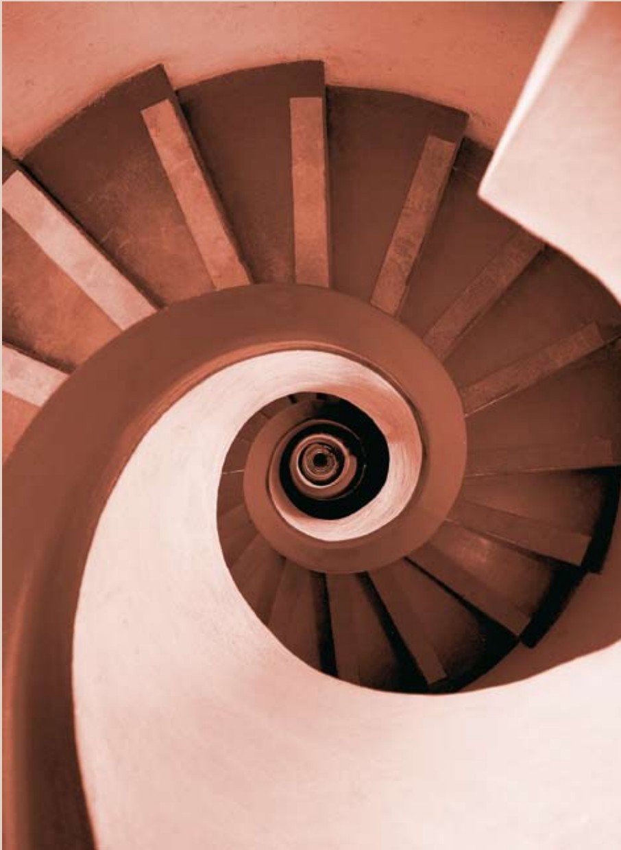
The 115-foot Caracol tower has no elevators and only enough space to walk in a single file line. In order to remove the boxes from the damaged tower, the staff, carrying one box at a time, had to ascend and descend the 160-step spiral case shown here.
