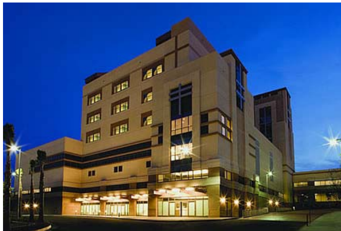
WMMC New Building
