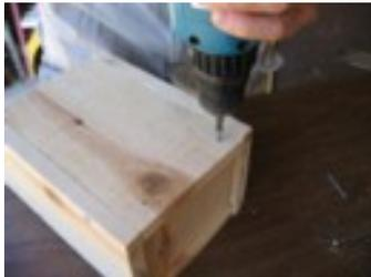
place. Pre-drill the holes and secure with six screws, each placed about 1 1/4" from the edges of the house, two from the front, two from the back and two from the stationary side. Make sure you don't put any screws through the opening
