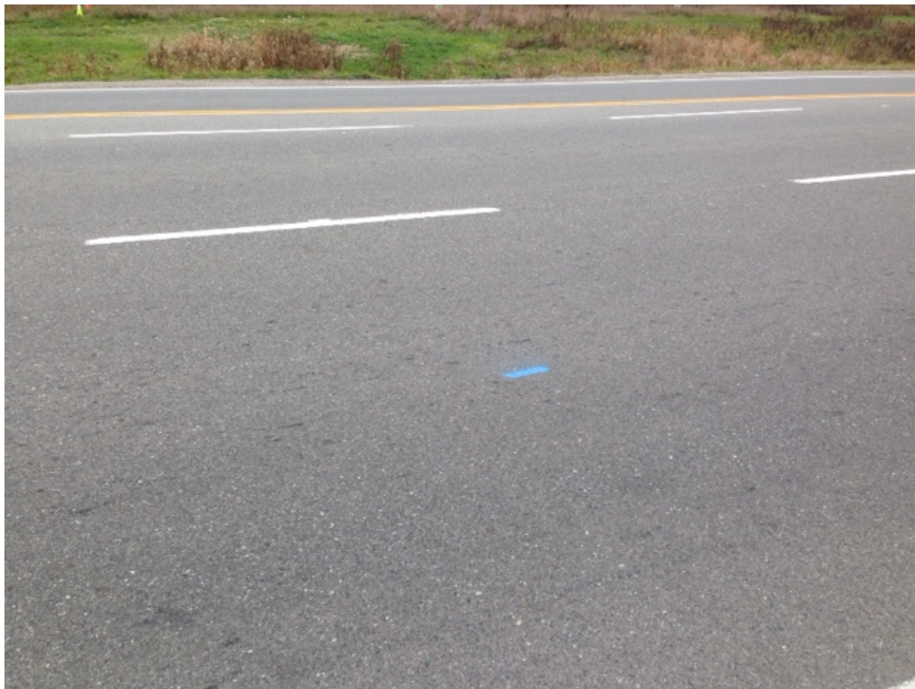
Photograph 2: Looking across lanes of Section 1.
