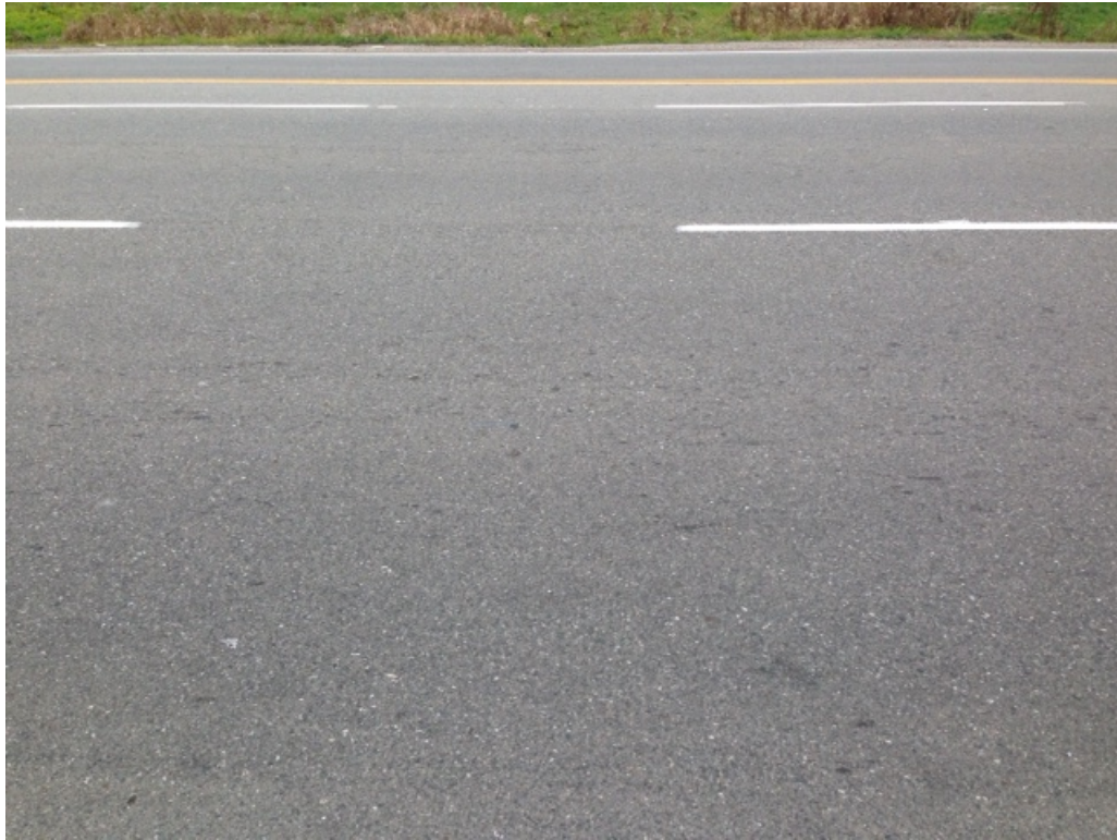
Photograph 3: General pavement condition along Section 1.
