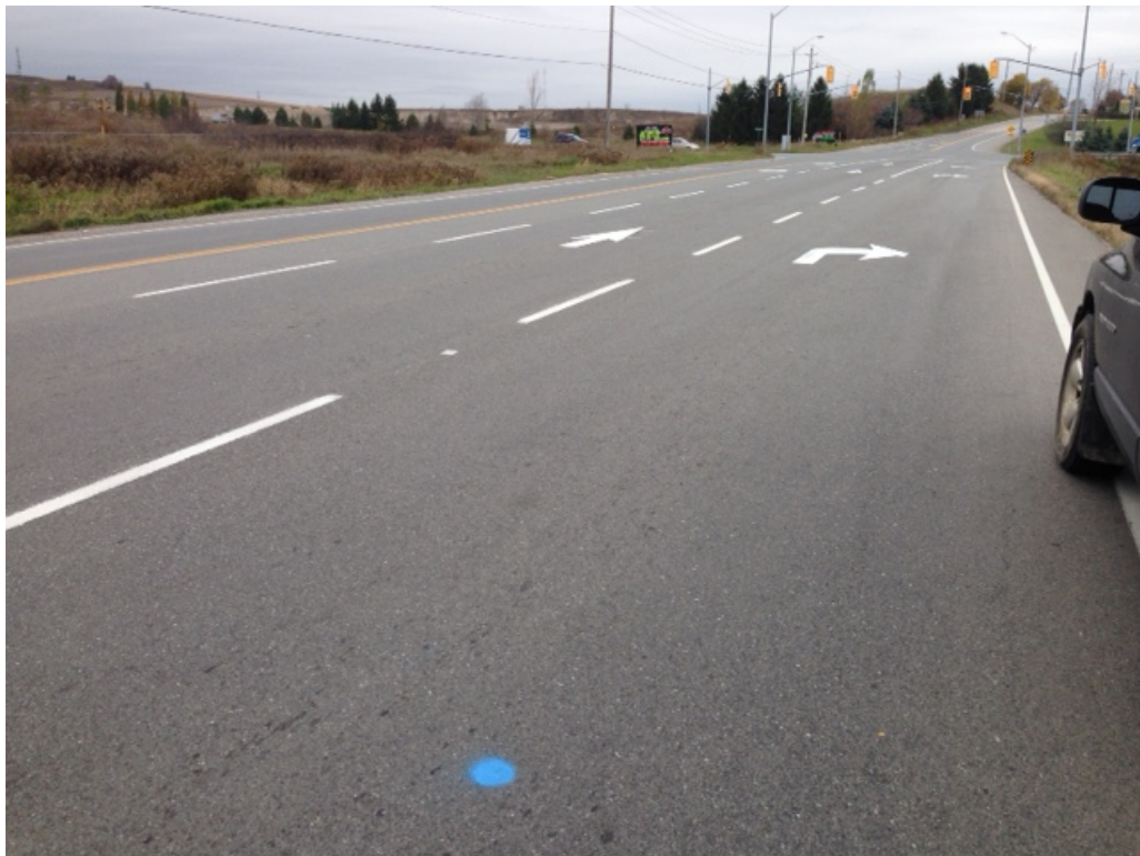
Photograph 4: Looking north on Section 1.
