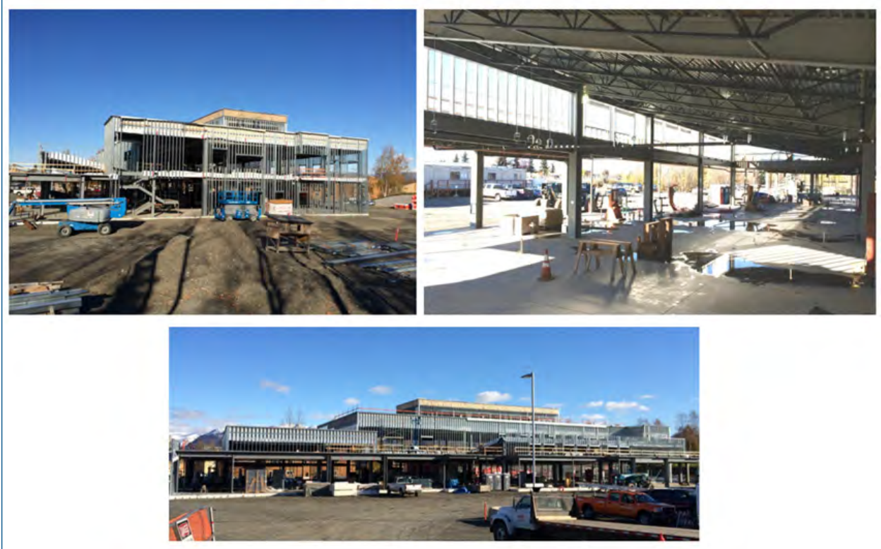
Photos 1-3. Construction Photos
