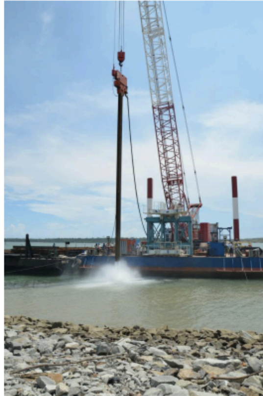
Toyo Simba drives the first steel pipe pile.
