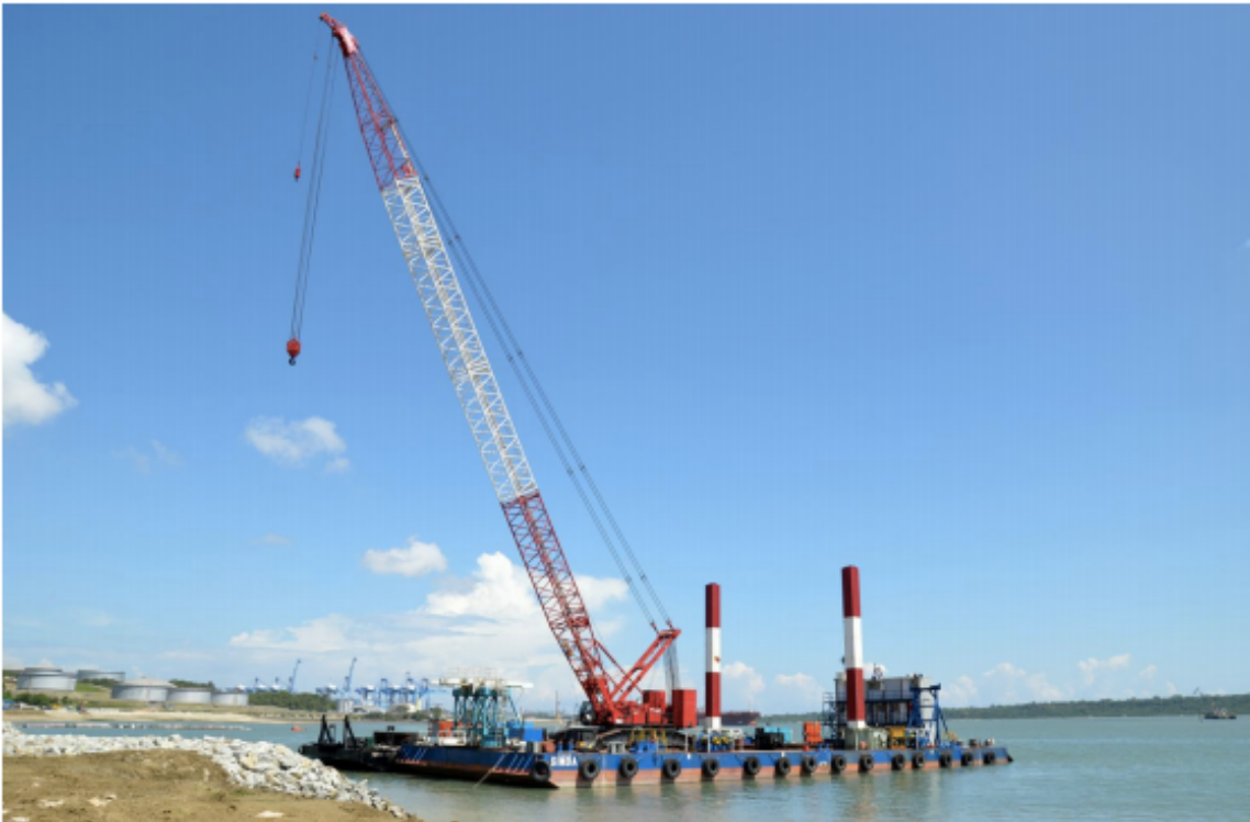
Toyo Construction's pile-driver and crane ship, Toyo Simba
