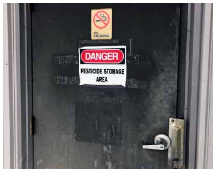
Store pesticides in a lockable concrete or metal building separate from other buildings. Photo credit: John McMullan.
