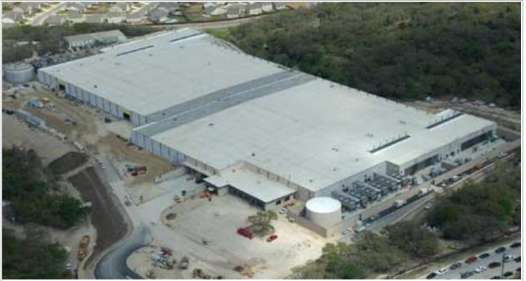
An aerial view of the 470,000 square foot Microsoft data center in San Antonio.
