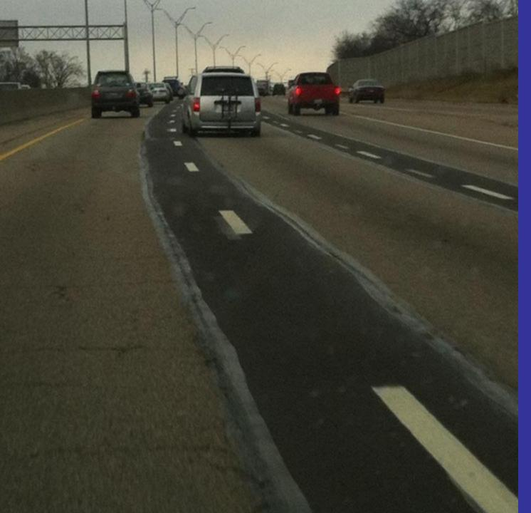
I-71 in Columbus " In recent years, it has become evident how critical longitudinal joint construction is to the life of the pavement structure...
