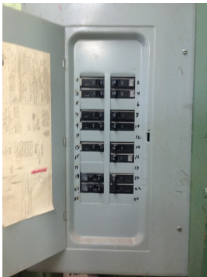
Figure 18. The Service Entrance Panel (SEP) and sub-panels house the circuit breakers for the AC circuits.
