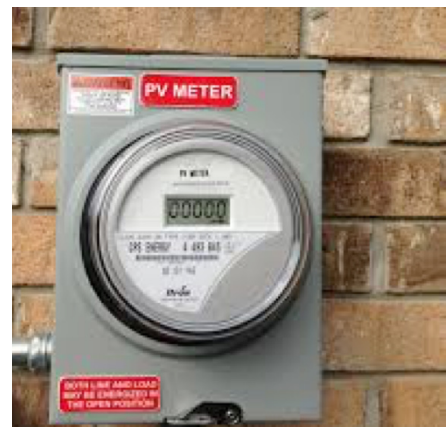
Figure 19 Example of meters used to monitor system performance including battery-bank charging, and energy (kWh) production of a PV system.
