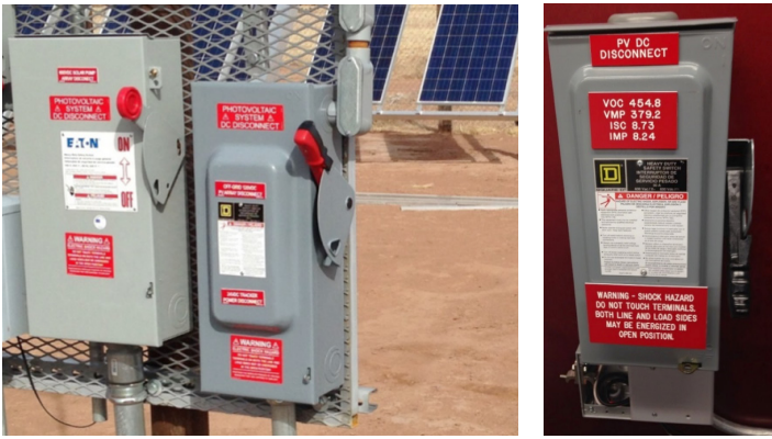
Figure 7. Examples of DC safety disconnect switch boxes. The one on the left is part of an active solar array. The box is properly labeled as a PV DC disconnect switch with the amount of energy coming through it.
