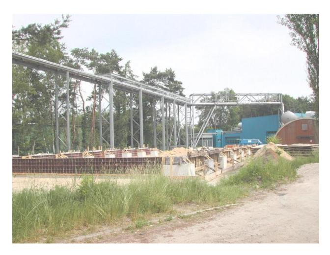
4.5 K and thermal shield flow from HERA cryo-plants to TTF
