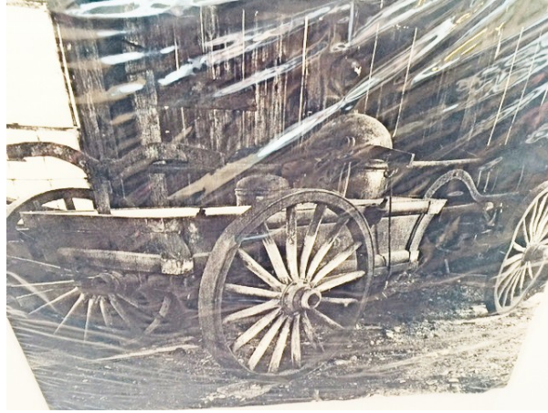
Neptune Pumper Showing Damage From 1910 Fire.
