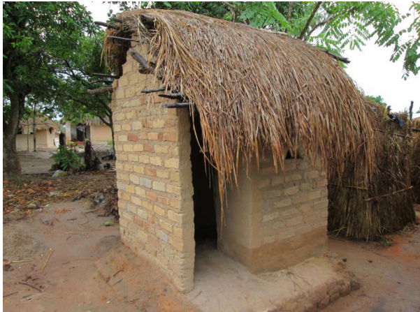
Figure 4: Tiny latrine with narrow entrance
