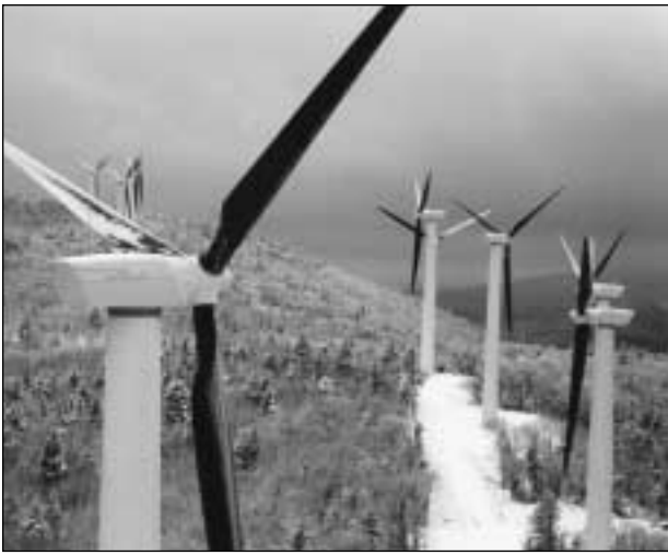
The 6-MW Green Mountain power plant in Searsburg, Vermont, consists of eleven 550-kW wind turbines.
