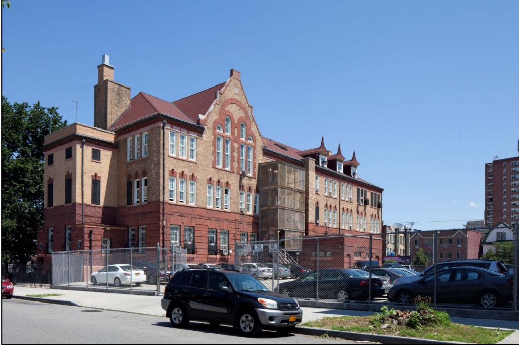
Jamaica High School (now Jamaica Learning Center) Views of rear of building Photos: Christopher D. Brazee, 2013
