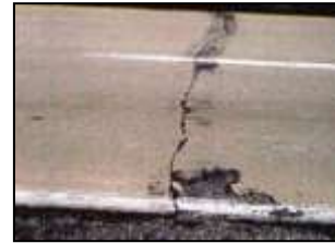
Bottom up & Top Down Cracking (JPCP Only)
