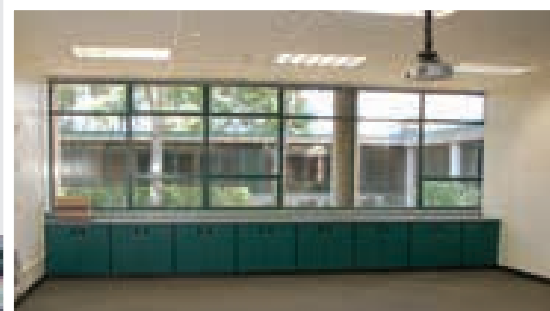
One of the old biology labs in Upper Arrupe was split in half to create two classrooms that will be utilized primarily for English classes. The new classrooms are now Rooms 40 and 41.
