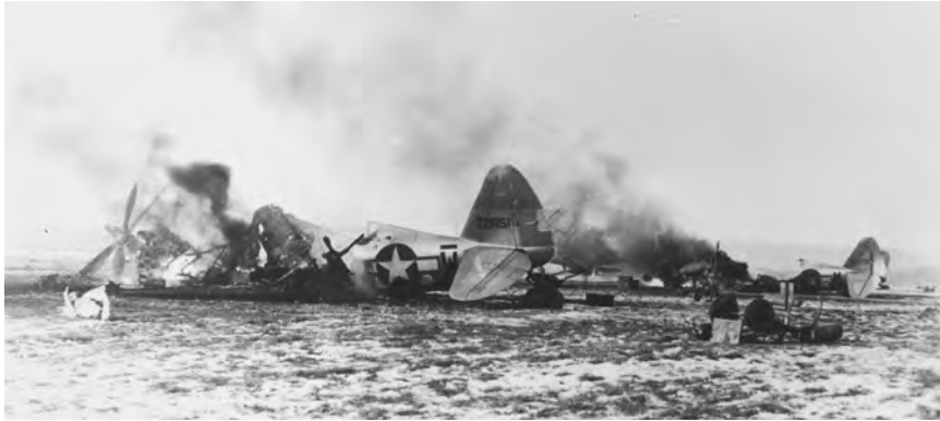
Damage caused by the Luftwaffe raid on January 1, 1945
