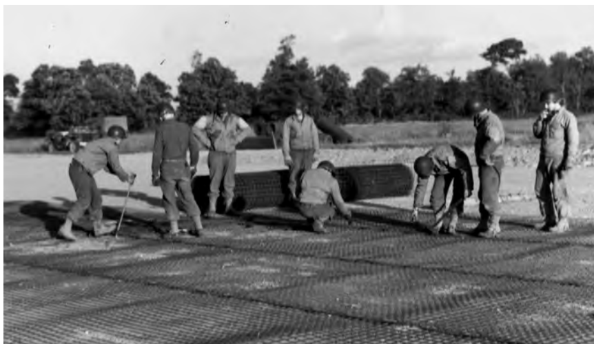
Army engineers handled airfield construction and maintenance for Weyland's advancing aircraft squadrons, laying steel mesh for emergency landing strips (top), and on occasion broom-massaging the airstrips (bottom).
