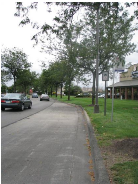
Figure 6-20 Undesirable Bus Bay Design without Pedestrian Features
