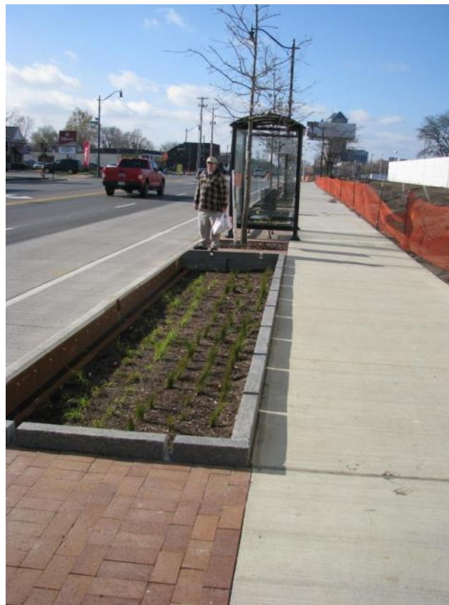
Figure 6-19 Bio-Swale Placed in Bus Passenger Alighting Area
