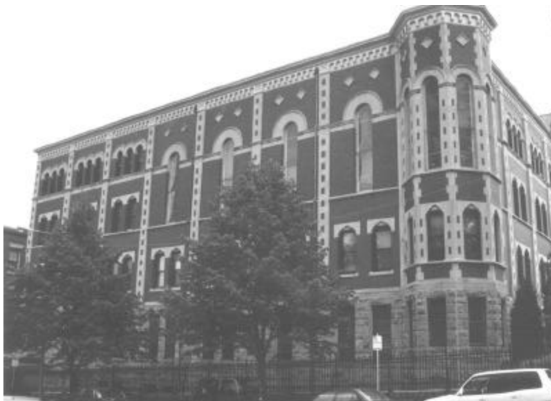
The rectory building from the corner of Tremont Street and St. Alphonsus Street
