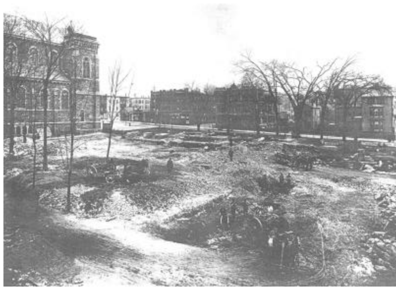
Construction of the rectory building
