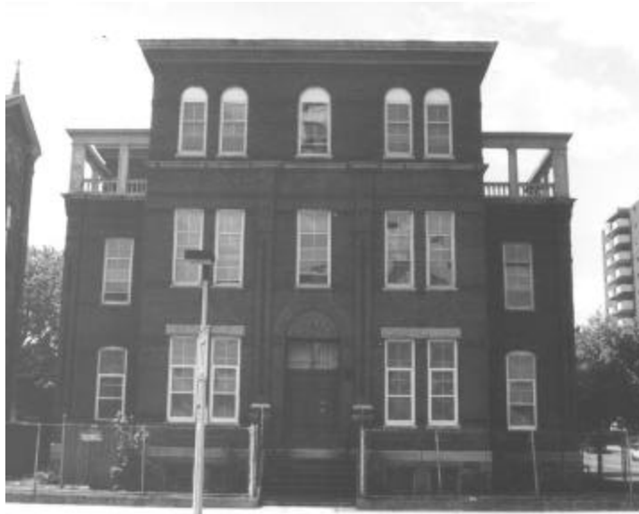
Front façade of the convent building (Smith Street)
